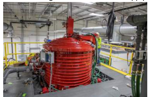
The Multi-Zone Direct Cast Vacuum Induction Melt Furnace at the Testing and Demonstration Facility
