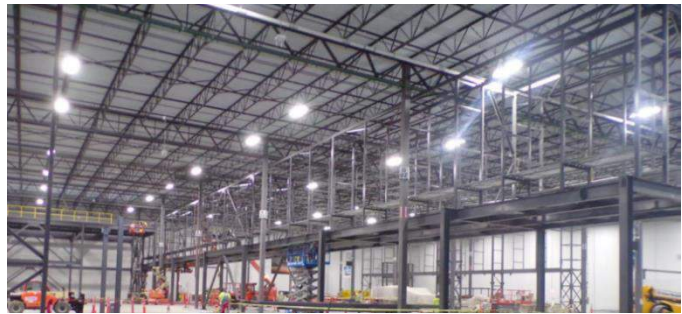
KC STEP Construction Initiated, and Occupancy Contracts Awarded
