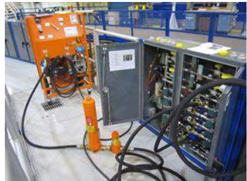
Sulfur hexafluoride reclaiming system being used on SNL's Z
