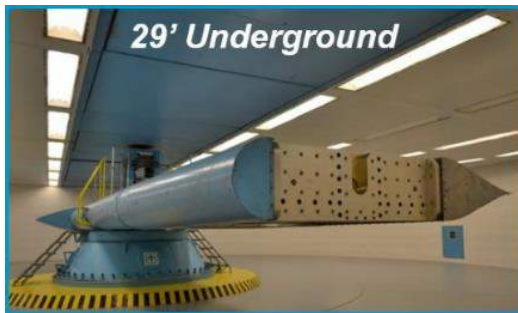
New Centrifuge Cooling System, Major Environmental Test Facilities, SNL
