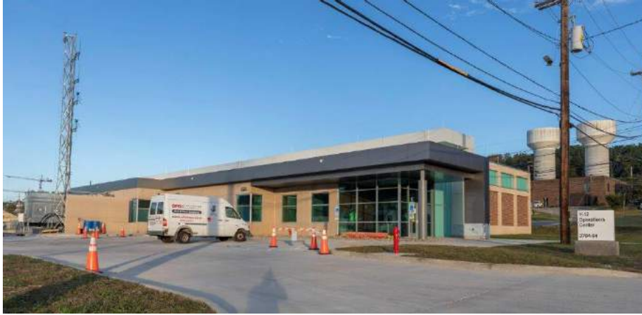
Construction at the Emergency Operations Center at Y-12
