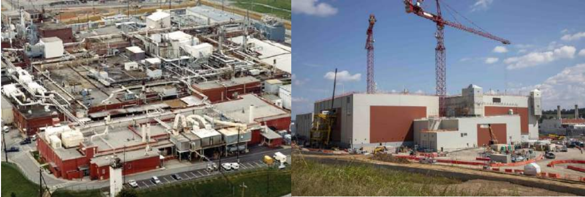
Manhattan Project-era Building 9212 at Y-12 (left) and construction on its replacement, the Uranium Processing Facility, in September 2022 (right)
