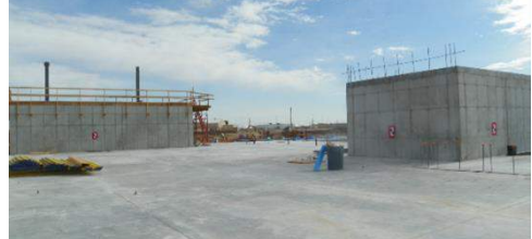
HESE HE Lab Blast Tank Pit Concrete Forming
