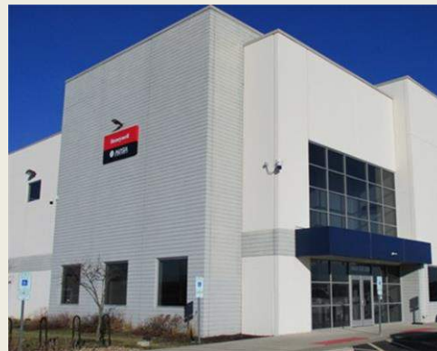
KCNSC East Building
