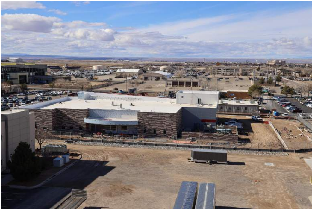
Construction on SNL's Emergency Operations Center
